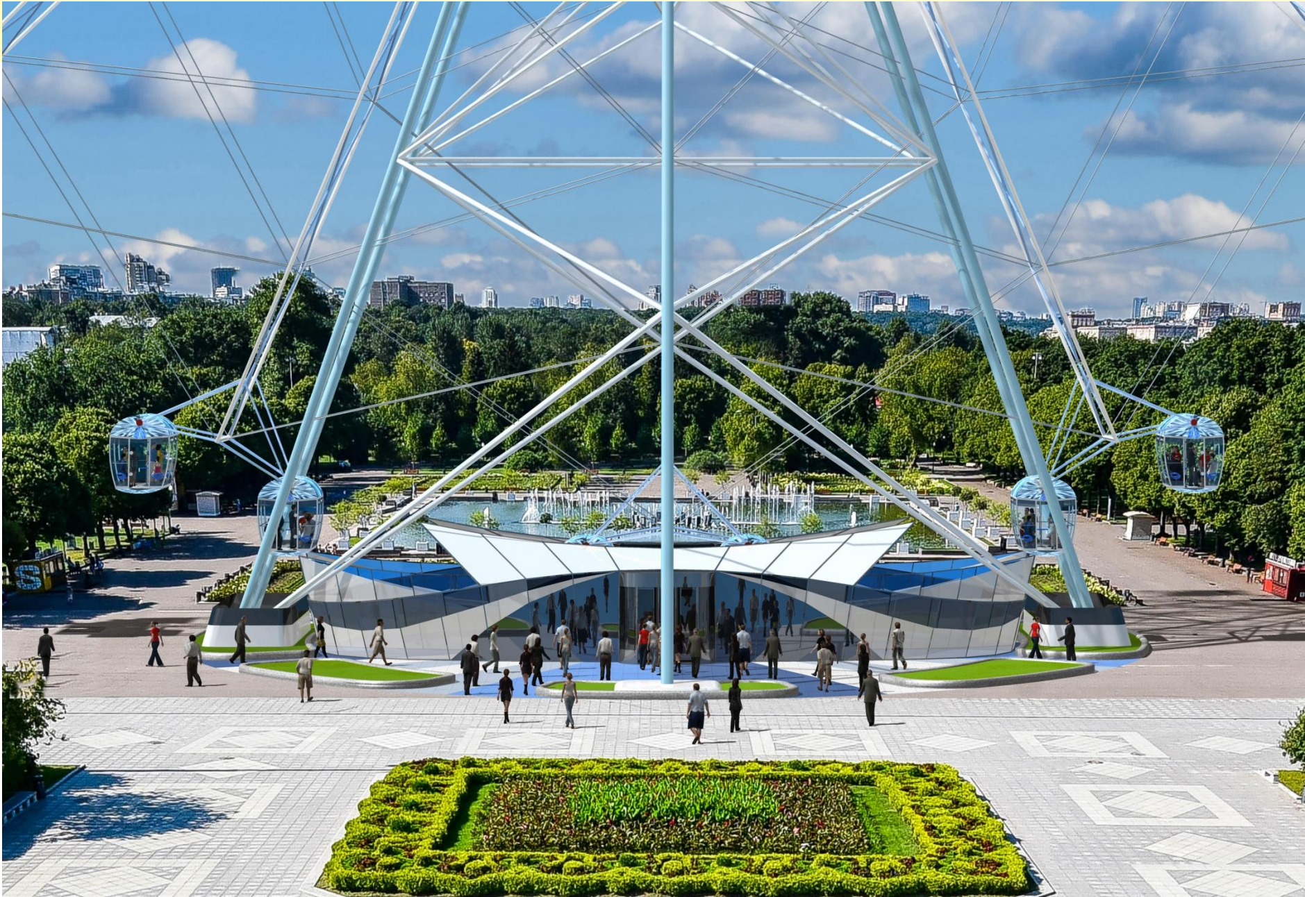
Station of a wheel 105-91m
