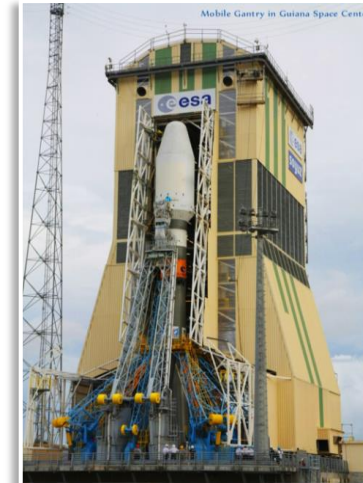
Mobile Gantry in GSC
